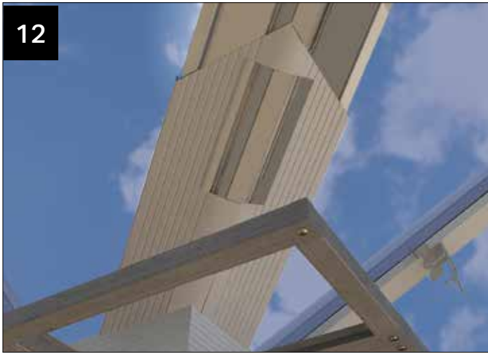
Fit the valley plate CHA016 (refer to steps 1-5, valley standard classic).
